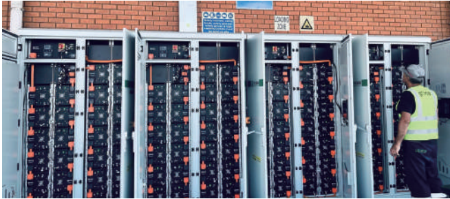
Renon AC ECube 186 kWh
