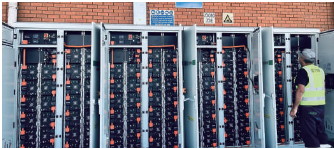
Renon AC ECube 186kWh
